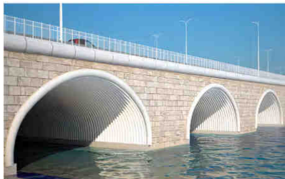
Fig. 1. Example of Multi-span Soil steel composite structure [5].
