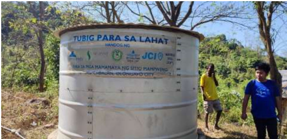
Figure 1. Initial Inspection of the Water Tank with the Chieftain (Photo credit to Mr. Kristoffer Paul C. Obispo)
