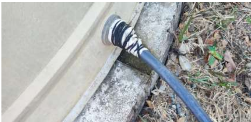
Figure 6. The Water Outlet Alternative Fix (Photo credit to Mr. Kristoffer Paul C. Obispo)
